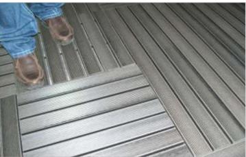
WPC does not decay internally, rot or propagate mold. It can be cut, drilled, nailed and sanded like normal wood. All these precessing can be done with standard tools. WPC flooring, lumber, cladding can be directly used untreated. WPC production is a 100% safe manufacturing practice having no process waste of materials, as production waste can be easily ground up and processed into top quality product again.
